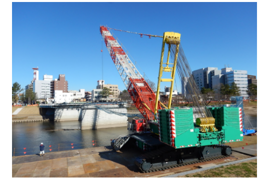
(仮称)乙川人道橋:架設状況(P1橋脚~P2橋脚)
